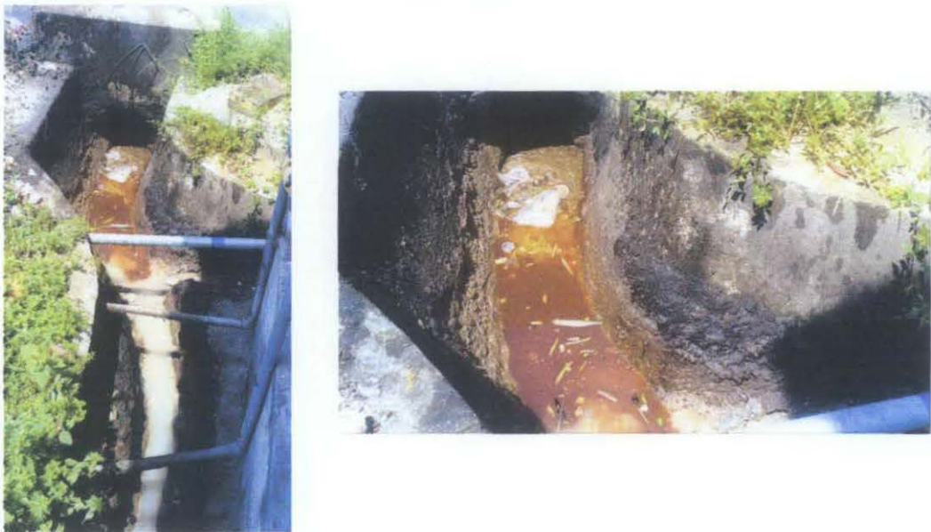
Figure 1.1: Discharge of Oily Restaurant Wastewater
