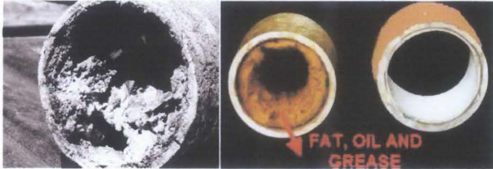
Figure 1.2: FOG deposits in sewer pipes (Stop the clog, n.d.)
