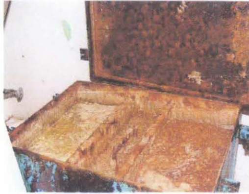
Figure 1.3: Kitchen Grease Trap/Interceptor (Blu Sky Biofuels, 2008)
