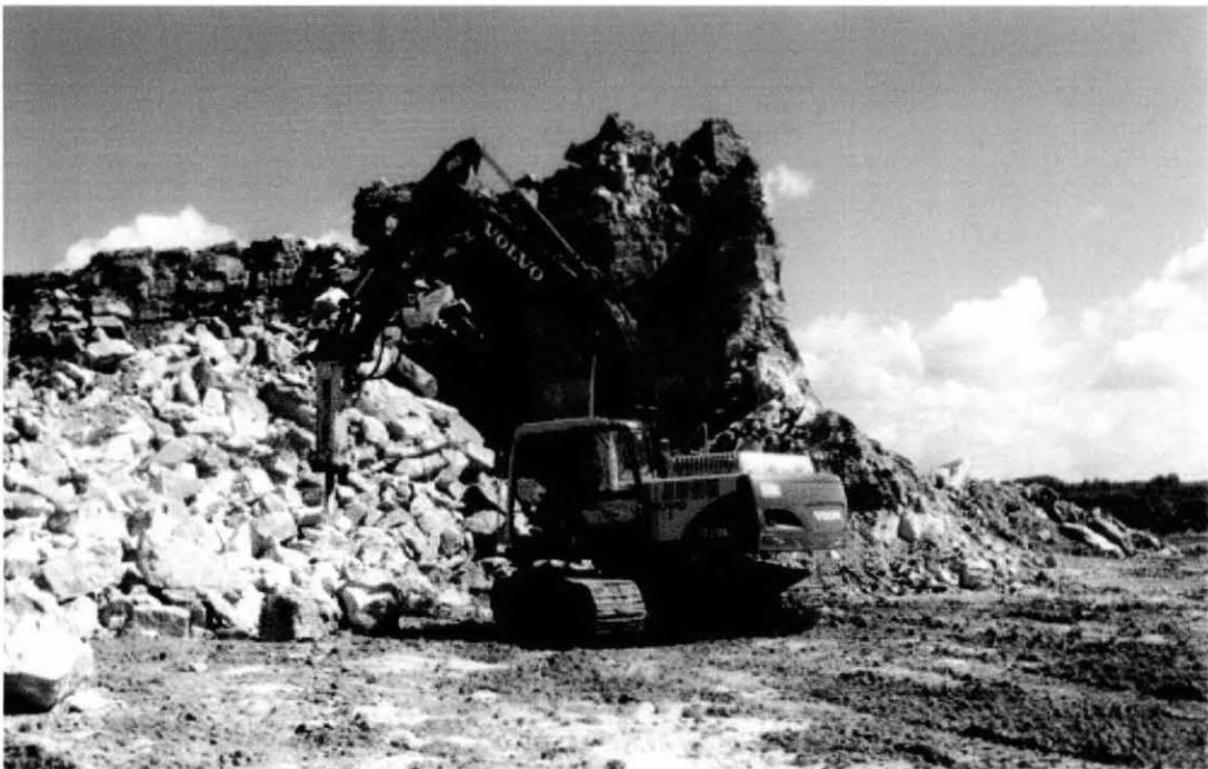
Figure 1: limestone blocks taken away for crushing
