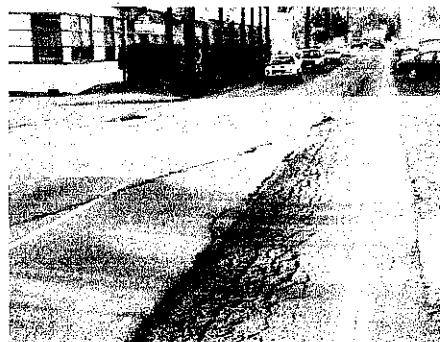
Figure 1.2: Rutting in pavement
