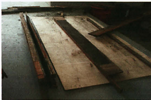
Figure 3.1: Ply wood and used form work from previous castings reused to construct the form work of required dimension to avoid wastage.
