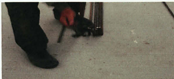
Figure 3.6: Steel Reinforcement bar bending activity (Y10 and Y12). Bars are bent about 3.5''
