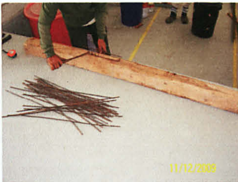
Figure 3.5: Bending of R6 links ( \Phi 6\text{mm} ) with dimension 3'' \times 11'' or 76\text{mm} \times 280\text{mm} .
