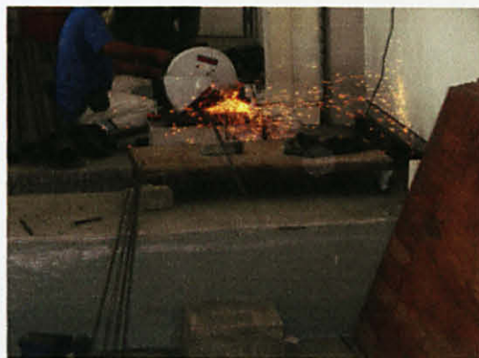
Figure 3.3: Cutting of steel reinforcement bars (Y10 and Y12)
