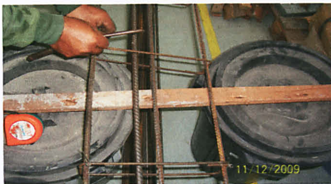
Figure 3.7: Tying of R6 links to main rebars Y10 (2 nos top bars) and Y12 (2nos bottom bar) using steel wires. The links are placed at a distance 300mm C/C and adjusted to avoid passing through section of opening. (Opening is located 100mm offset from concrete surface as the concrete cover was set to be 100mm.)
