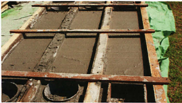
Figure 3.11: Concreted Beams to be cured for 2 weeks by using wet sacks to avoid rapid heat loss which could lead to cracking.
