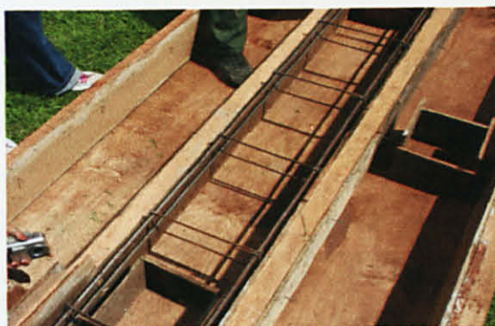
Figure 3.9: Placing Reinforcement bars into form work
