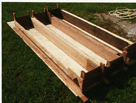
Figure 3.2: Completed form work of 3 beams to be casted on 1 ply wood.
