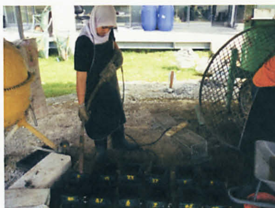
Figure 3.4 : Compaction using Vibrator
