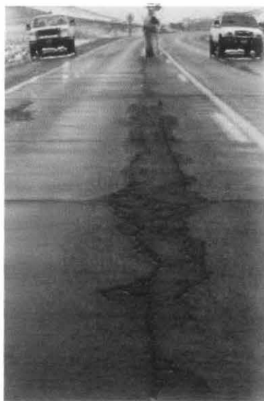
Figure 2.5 c: Stripping on pavement
