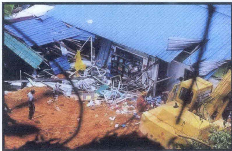
Figure 5: Landslide tragedy at Hulu Langat, Selangor [13]
