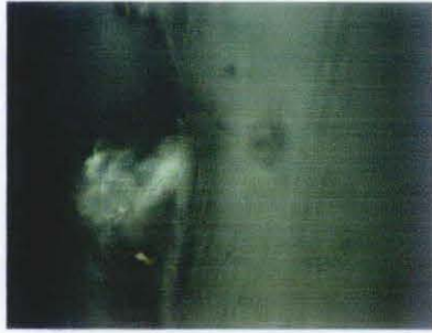
Figure 4.2: Presence of Delamination Observed at the Edge of Drilled Area using OM.
