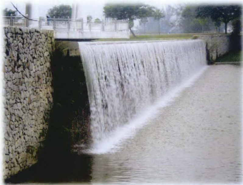
Figure 1.2: 3 metres water cascade at UTP mosque
