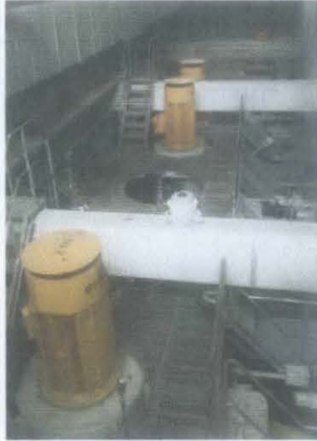
Figure 4.8 Sewage lift pumps
