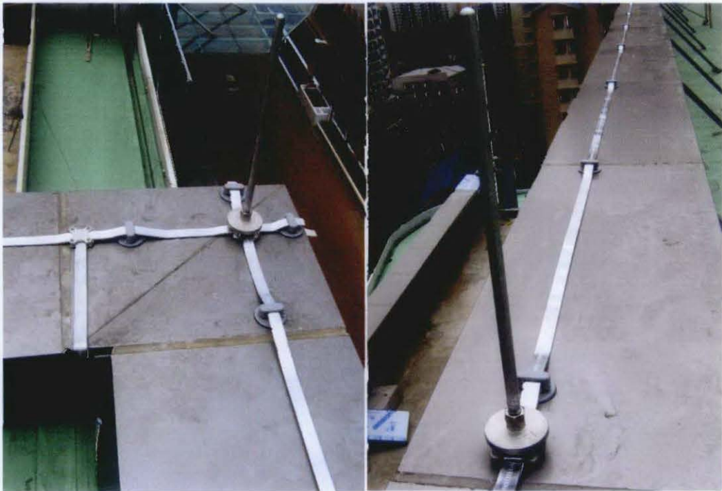
Figure 13 Proper bonding air terminal with copper tape at roof top [31]
