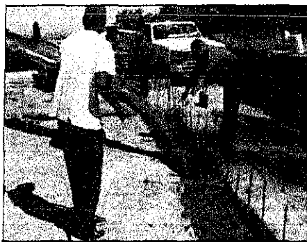
Figure 2.4: Placing of SCC
