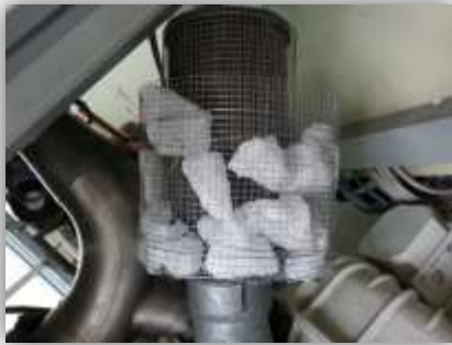
Figure 15: Inlet Air Cooling Method
