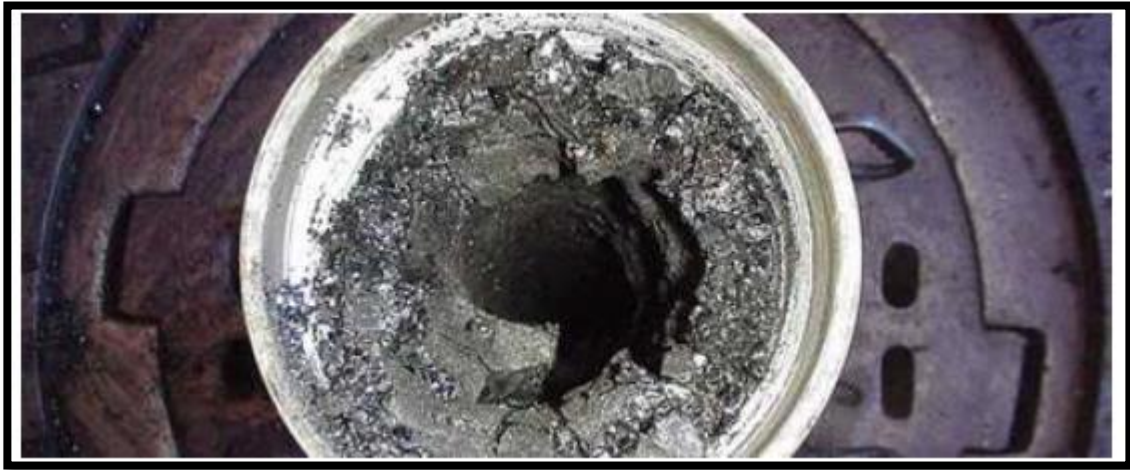
Figure 4: Asphaltene Precipitation in Pipe
