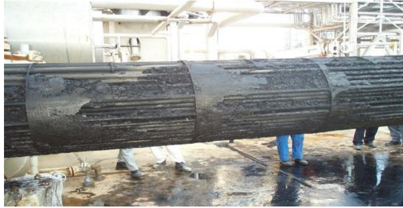
Figure 3 - Damaged separation facility equipment due to asphaltene deposits
