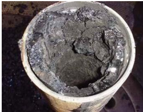
Figure 2 - Production Tubing with asphaltene precipitate
