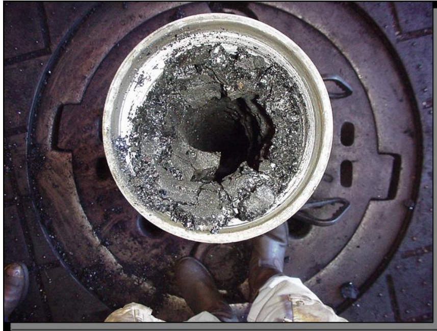
Figure 2: Asphaltenes deposit formed on the inside of a pipeline in a refinery (McKenna, 2009)
