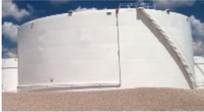
**Figure 24: Floating Roof Tank.**
