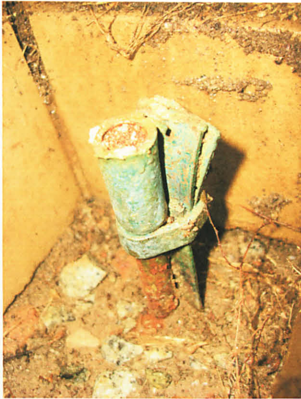
Figure 13 Copper Tape (right) Clamped To Copper Rod (left)
