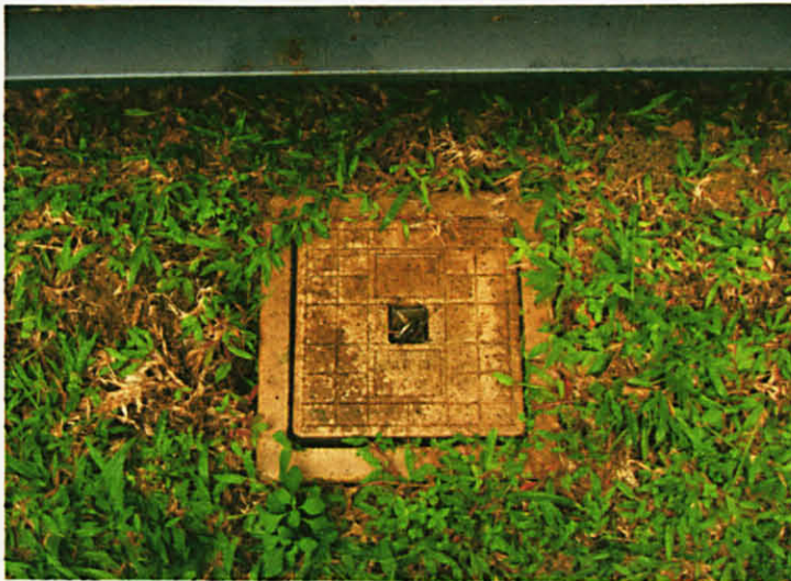
Figure 10 Overall View of An Earth Pit
