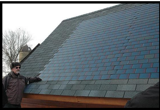
Figure 28: Dow powerhouse solar panel looks like ordinary roof shingles
