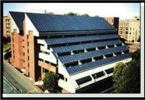
Figure 27: Example of Integrated Array mounting
