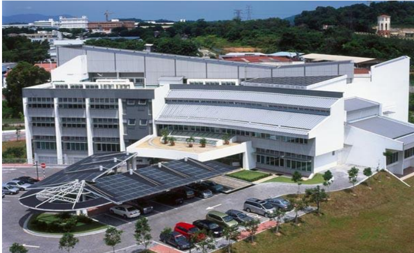
Figure 9: Aerial view of ZEO building
