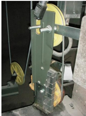
Figure 4.9: Machine Deviator Pulley
