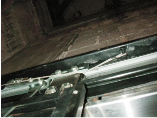
Figure 4.11: Suspension Roller & Track
