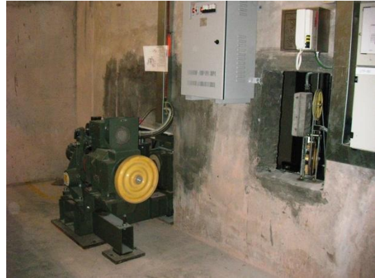
Figure 4.2: Gearbox & Pulleys
