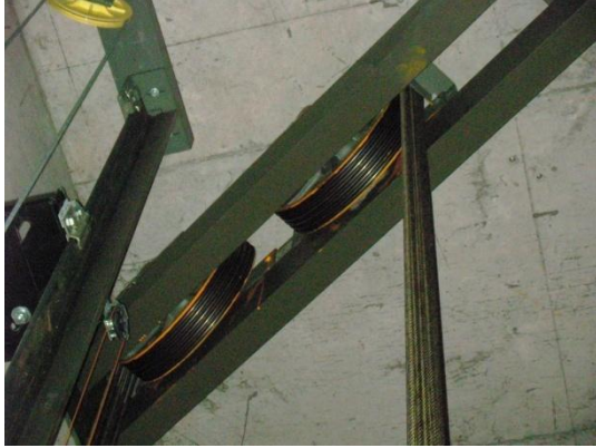
Figure 4.21: Pulley Top Shaft
