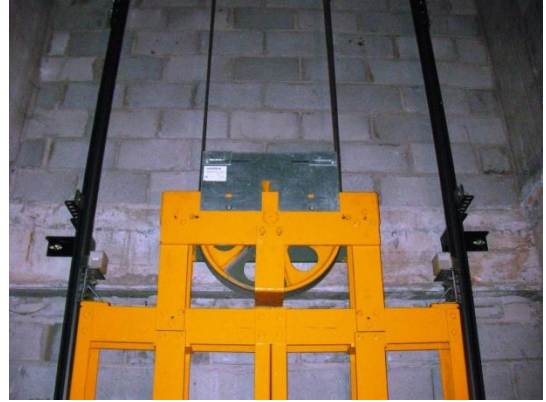
Figure 4.22: Counterweight
