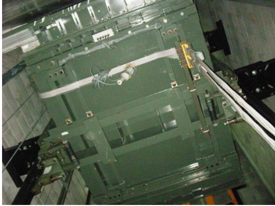
Figure 4.24: Bottom of Car
