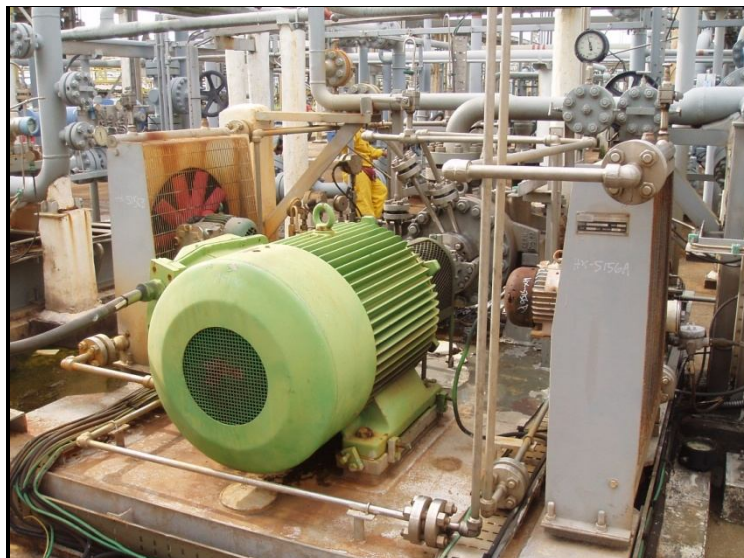
Figure 2.1: Condensate booster pump at OSC
