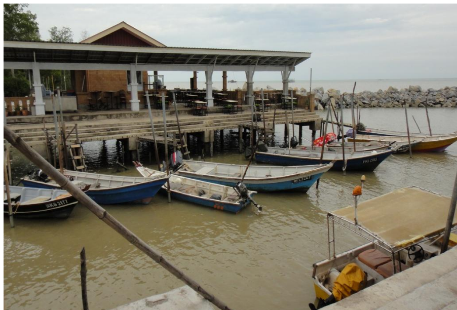
Figure 14 Jetty Pantai Siring
