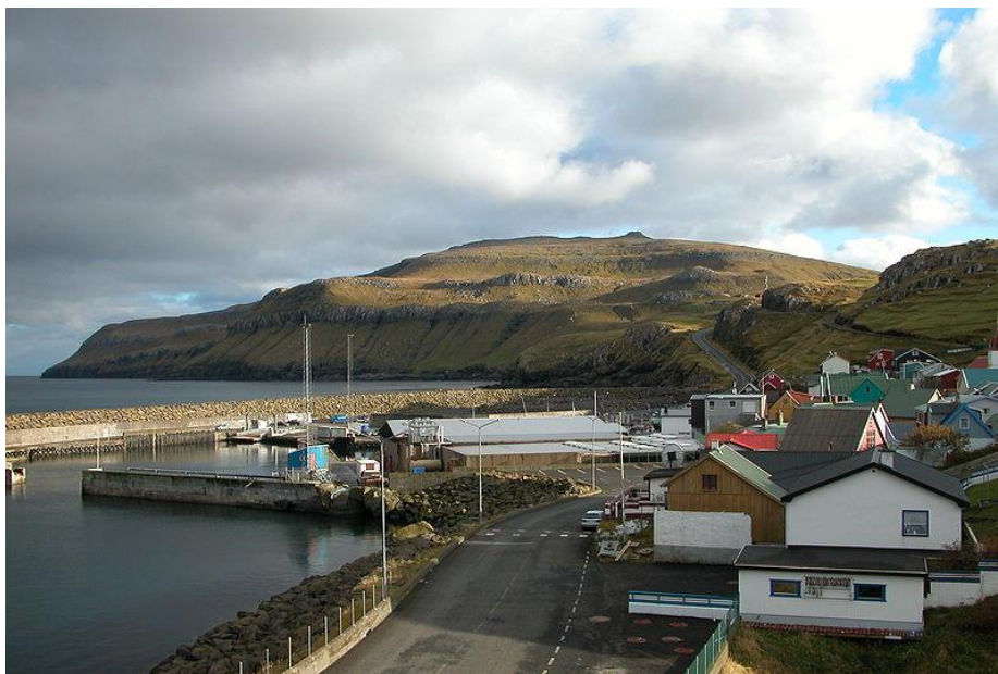
Figure 7 Skopun Berm Breakwater constructed in Faroe Island (Wikipedia, 2013)
