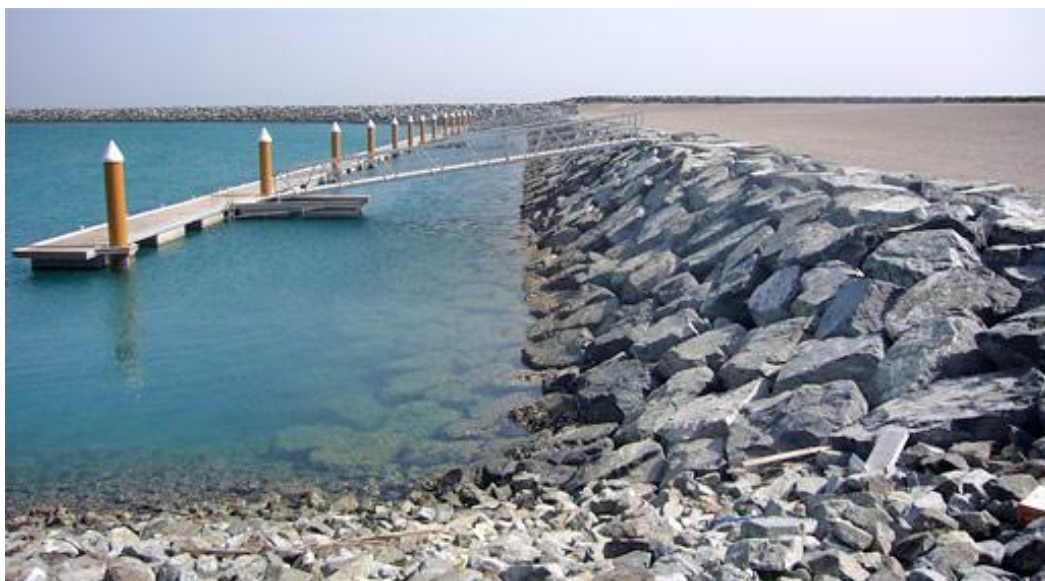
Figure 3 Rubble mound breakwaters constructed along the shoreline (Halcrow Corporation, 2011)
