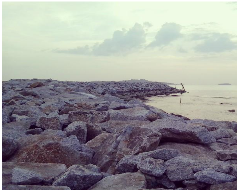
Figure 15 Segmented breakwater constructed at Jetty Pantai Siring
