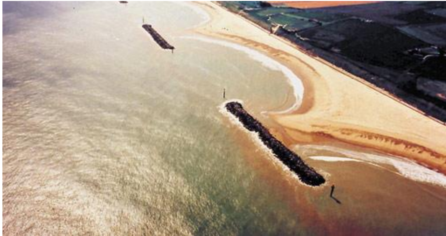
Figure 4 Rubble mound breakwaters constructed few meter shoreward (Halcrow Corporation, 2011)
