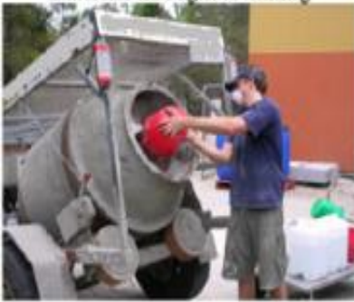
10-20min - Addition of fluid and dry materials throughout mixing
