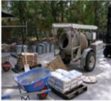
10-20min - Addition of fluid and dry materials throughout mixing
