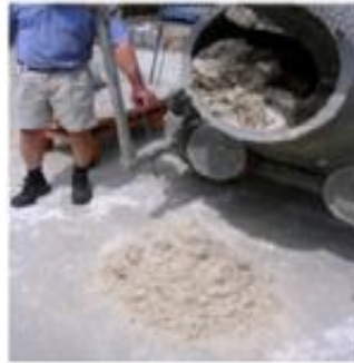
0-5min - Pre mixing of fine sand and steel fibres
