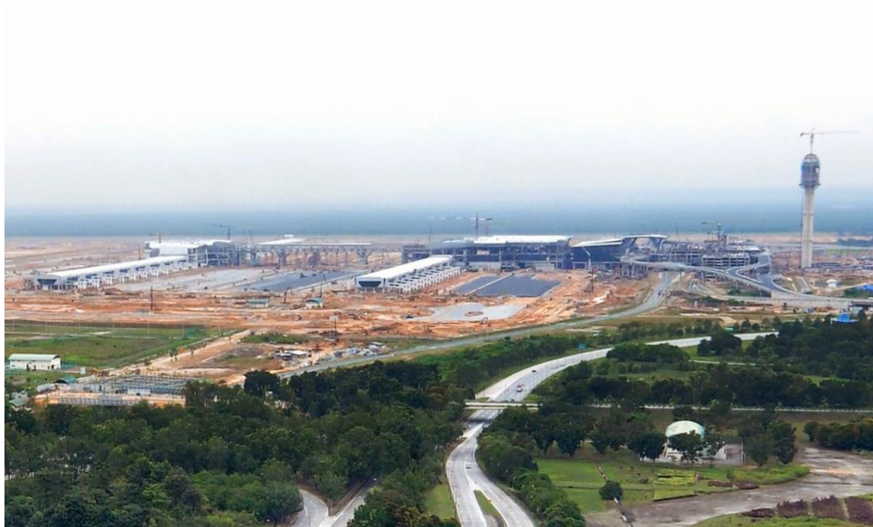
Figure 1.3: KLIA2 Construction Progress
