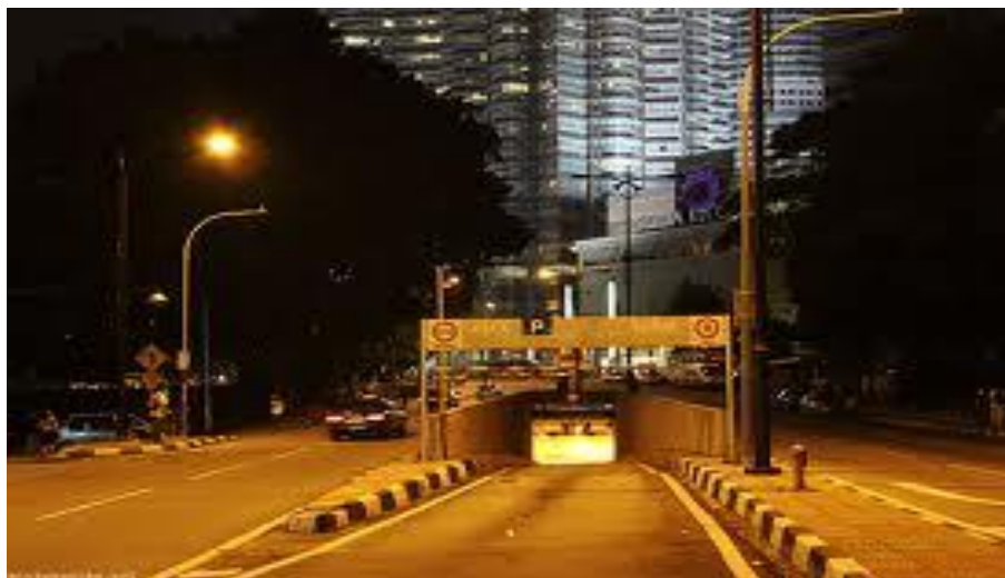
Figure 3: Ramp to the basement car park
