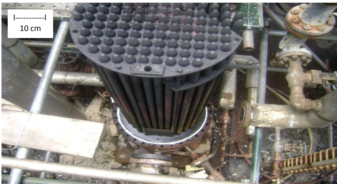
Appendix 2: Heat exchanger tube arrangement at the skid position
