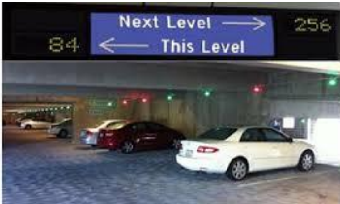
Figure 1: Example of Parking Guidance System
