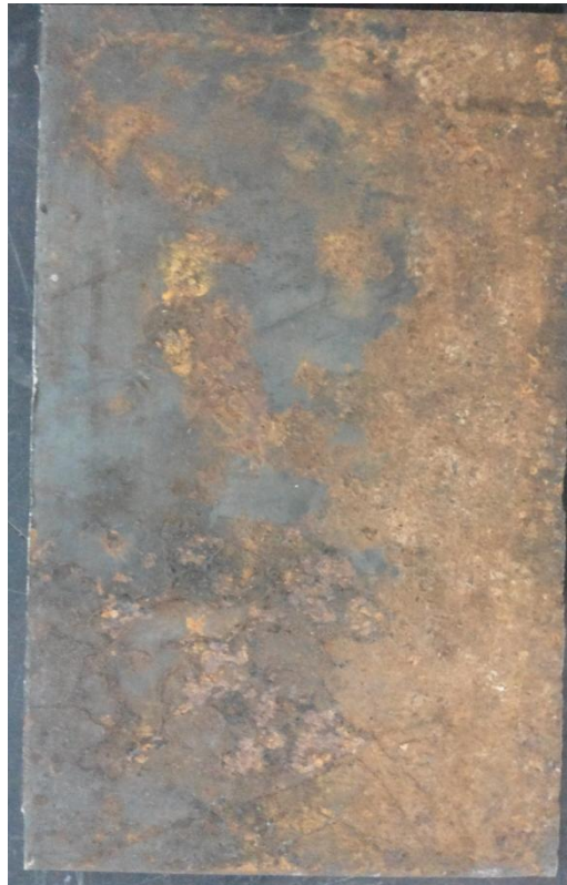
Figure 6. Steel after corrosion process has occur
