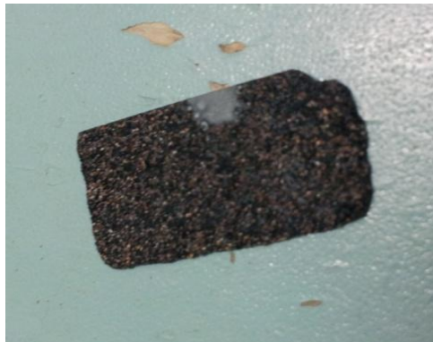
Figure 34 Front side of the coating layer where testing is carried out.
