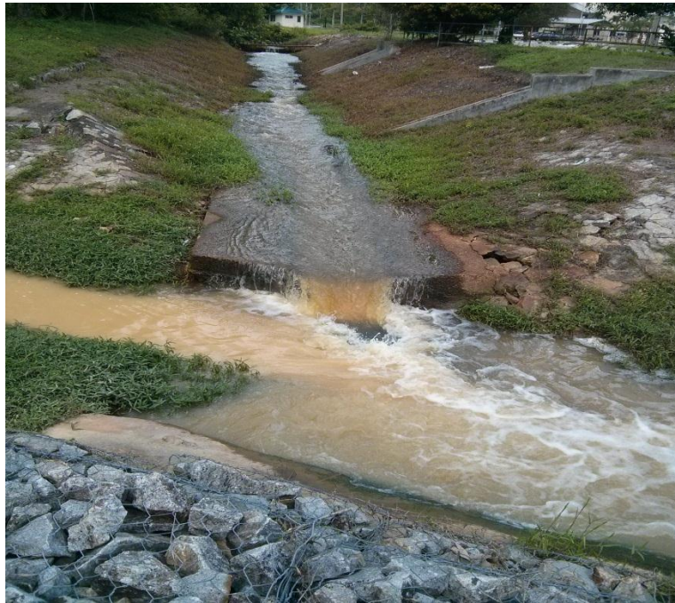
Figure 10: Picture of the hydro electrifier site before the dam is placed
