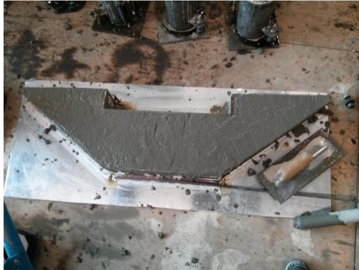
Figure 14: Concrete mixture is placed inside the foam work to shape the concrete
