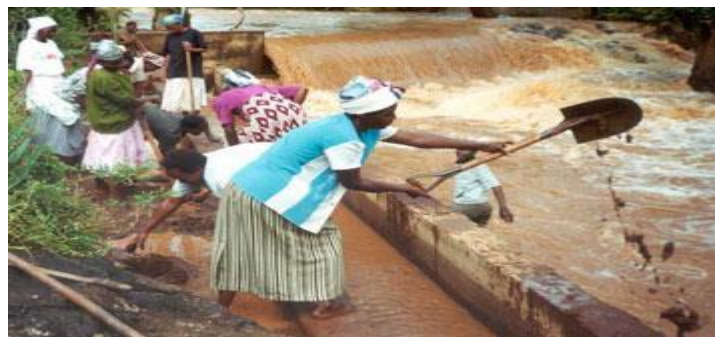
Figure 4: Clearing the canal for pico hydro power generation (Photo from Martin Wright/Ashden Awards, 2004)
