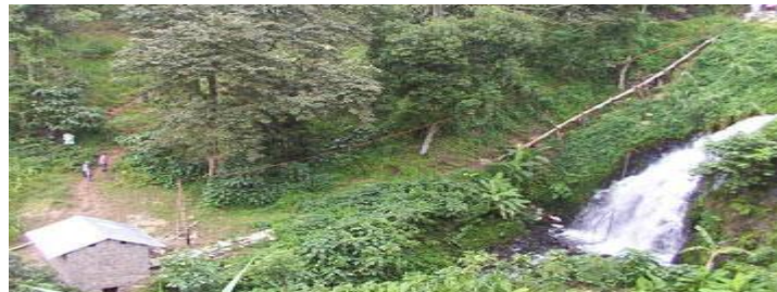
Figure 3: Power house for a pico-hydro power generation in Kenya (Photo from Martin Wright/Ashden Awards, 2004)
