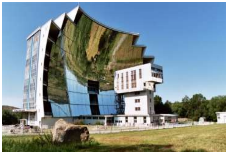
Figure 19: Solar Furnace at Odeillo, France-Spain border. One of the largest solar furnace in the world [37]
