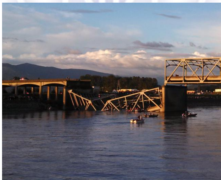
Figure 2: Collapse of Skagit River Bridge [5]
