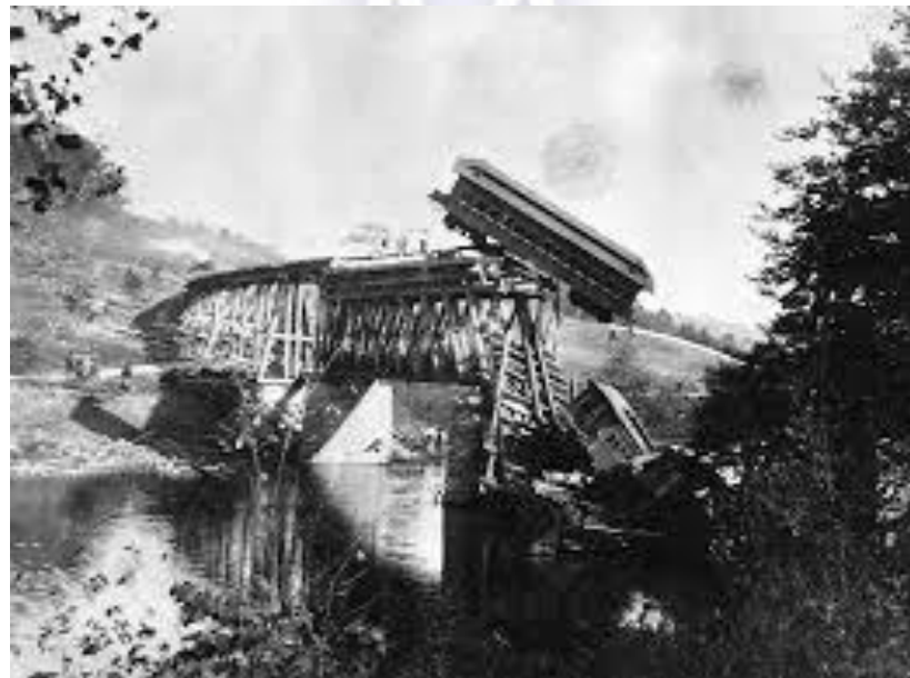
Figure 1: Collapse of Ashtabula River Railroad [4]
