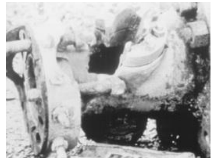
Figure 2.3: Surface choke failure (Courtesy of Baker Oil Tools)
