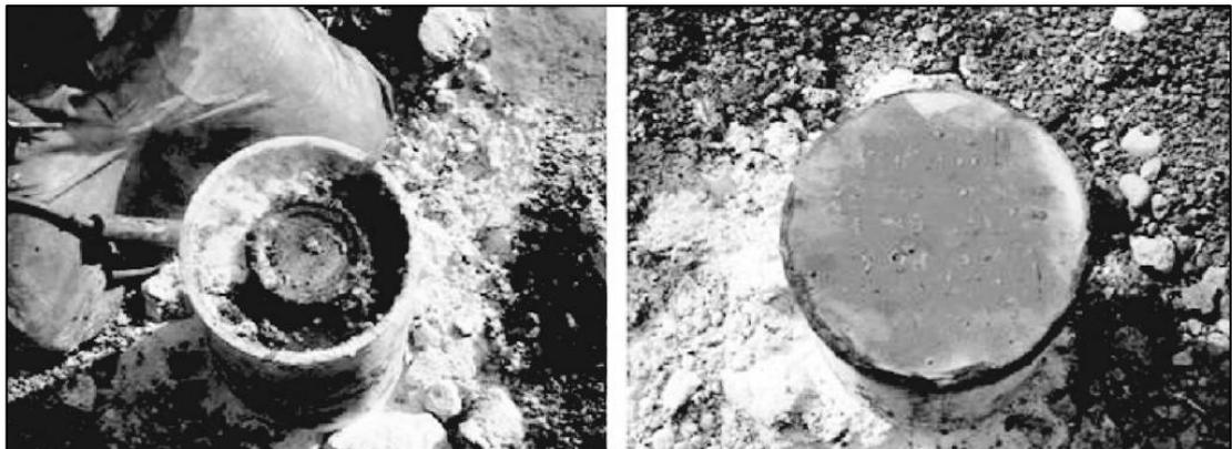
Figure 6: Wellbore cut and capped on production casing and surface casing [7]
