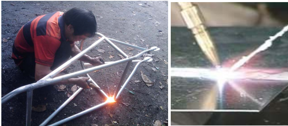
Figure 3.12: Aluminum welding using gas arc welding
