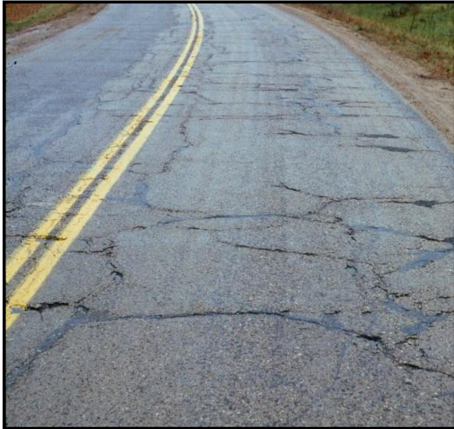
Figure 1.4: Block cracking
