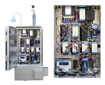
Figure 5: Aeroqual AQM60 Environmental Station
