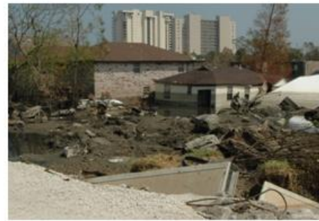
Collapse water defense system of New Orleans
