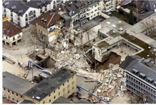
Train station building pit collapse, Köln
