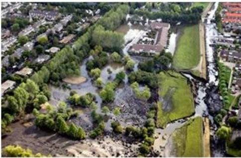
Peat dike failure, Wilnis
