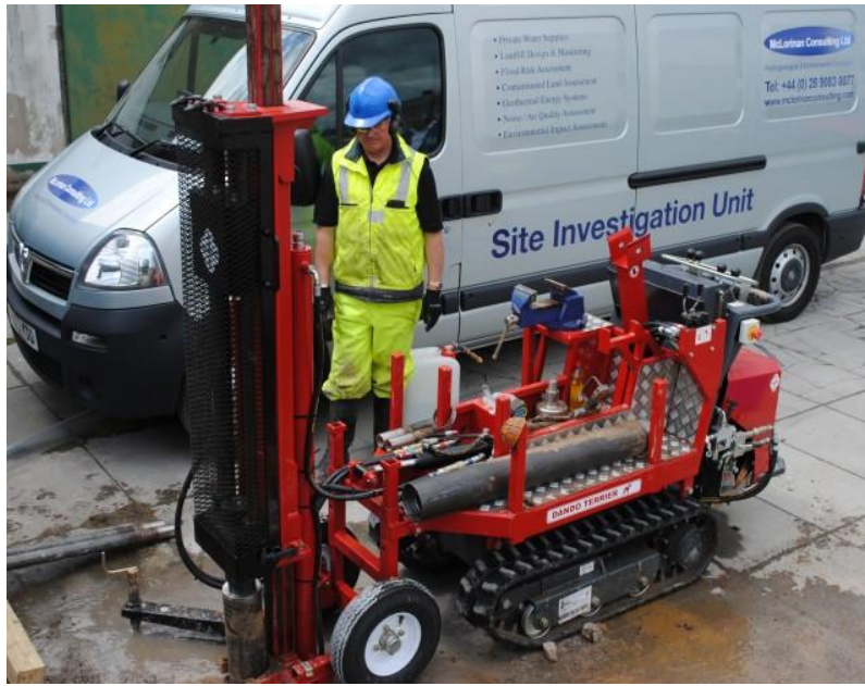
Figure 2.1.2 Common Borehole Sampling Procedure
