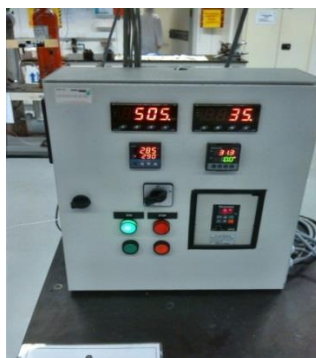
FIGURE 3.6 Autoclave Control Panel
