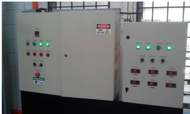
Figure 3.6: Starting system for MISEC
