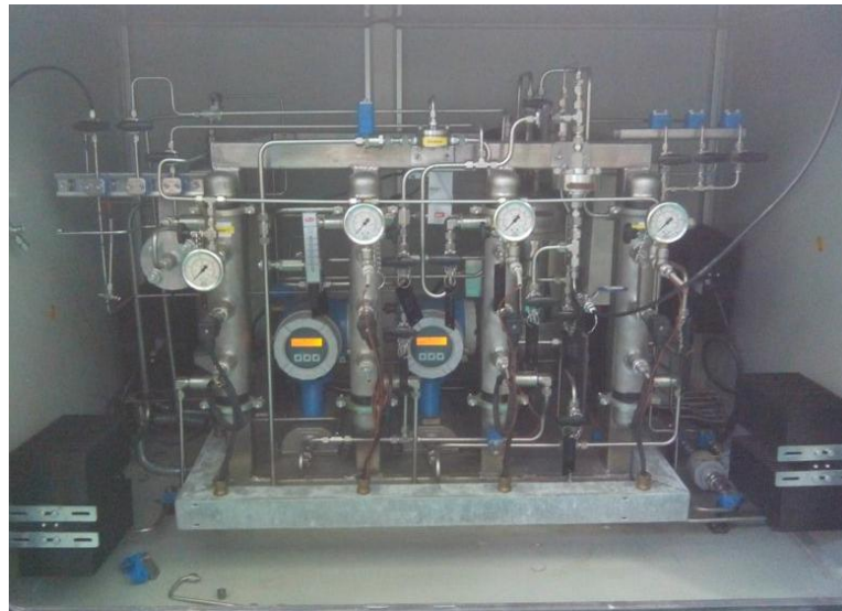
Figure 3.9: Monitoring pressure reading at the equipment
