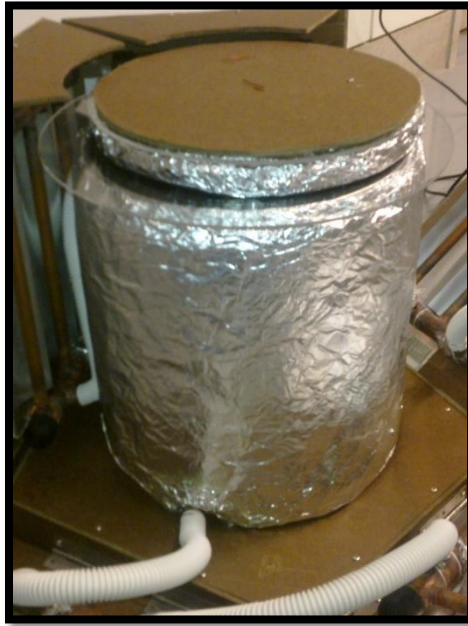
Figure 4.4: Hot Water Storage Tank
