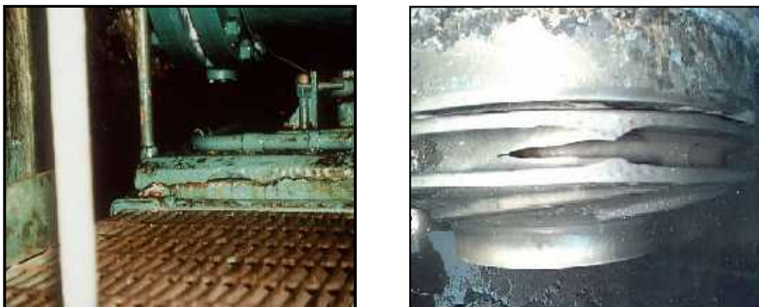
Figure 4 : Crack in Centrifugal Pumps
