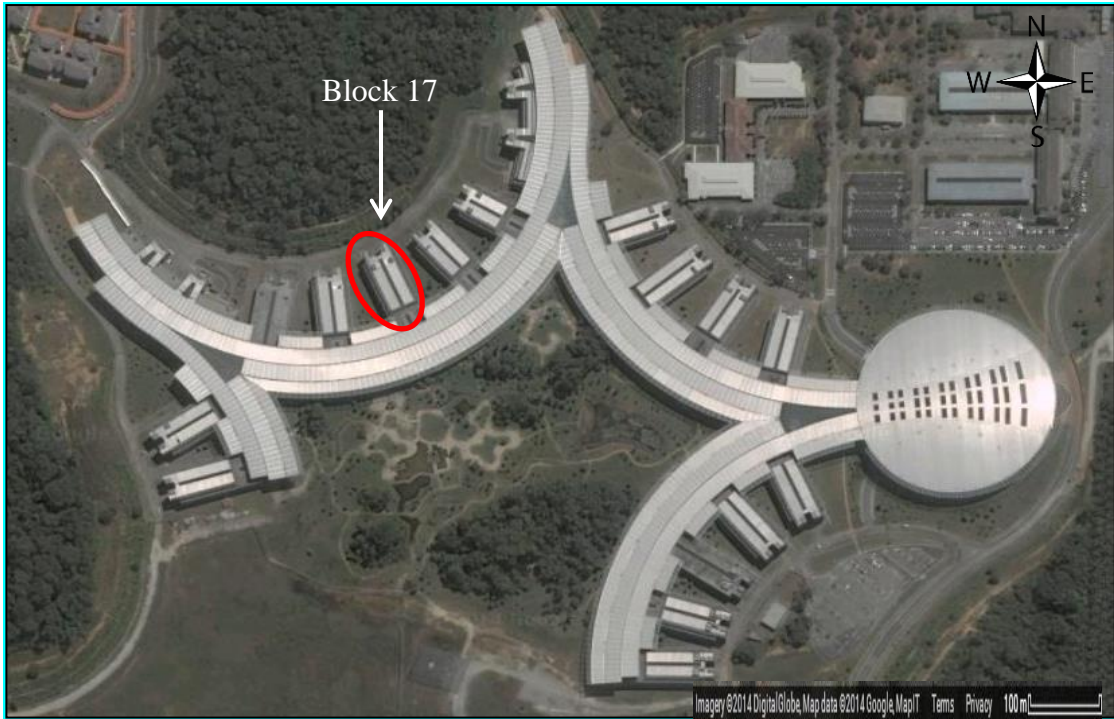
Figure 3.4 Location of installation at academic complex Block 17 (Google map, 2014)
