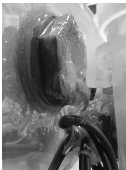
Figure 11: Hardened epoxy applied at the enclosure
