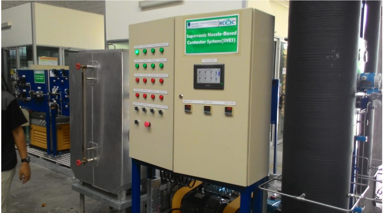
Appendix 6: Main control panel of the system
