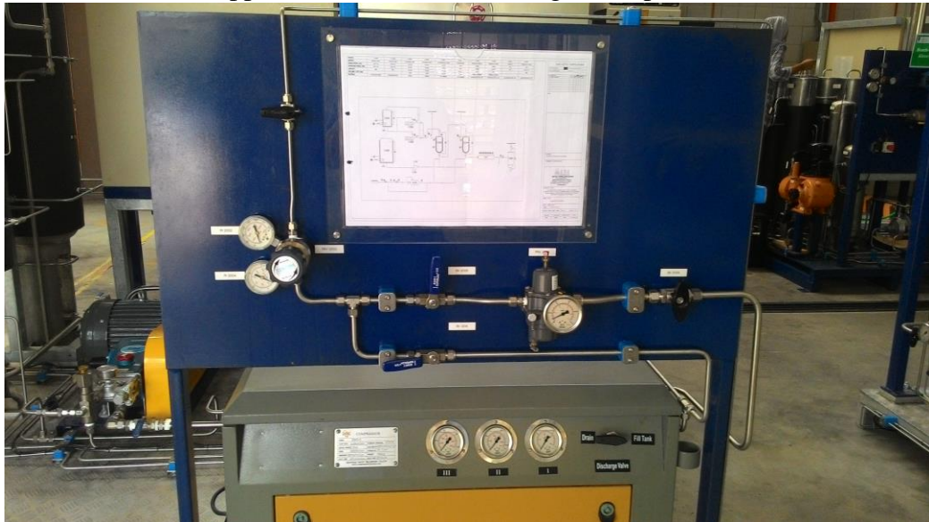
Appendix 5: Carbon Dioxide gas compressor
