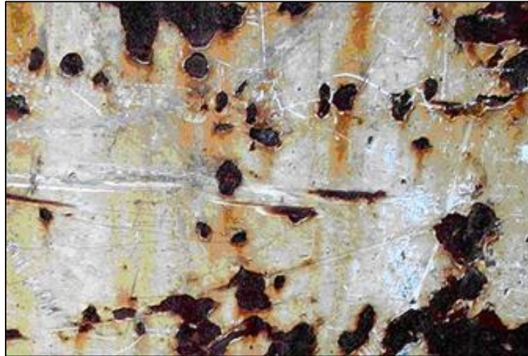
Figure 3: Delamination of paint cause by prolong exposure to moisture
