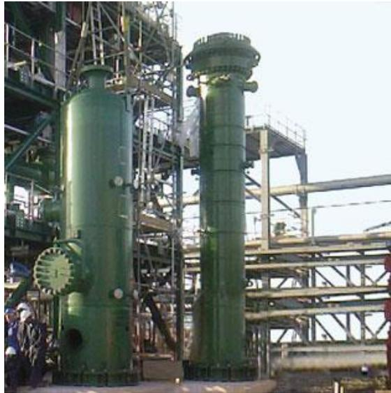
*Figure 2.3-2 Installed Hydrate Separator™ for JT-LTX system (TwisterBV, 2011).*
