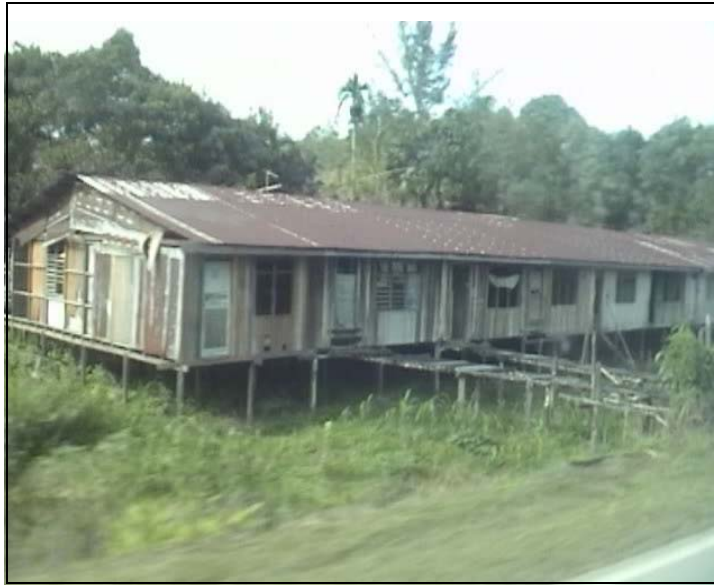
Figure 3: Corrosion of Metal Roofing in one of the rumah panjang in Sarawak
