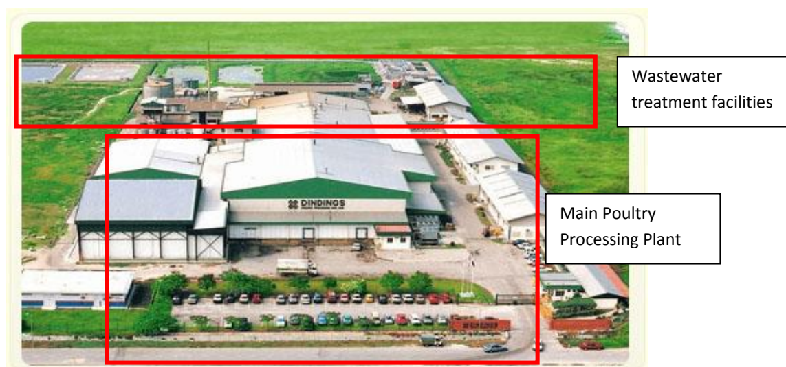
Figure 1- Dinding Poultry Processing Plant (DPPP) Sdn Bhd.
