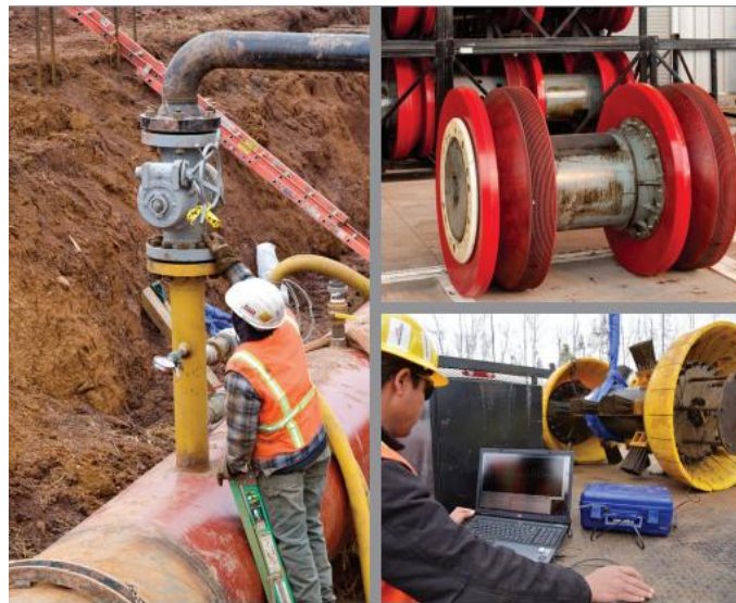
FIGURE 3: Hydrostatic Pressure Testing
